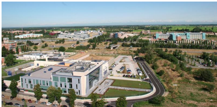
Figure 1 – Top view of the area occupied by CNAO. At the front the hospital building and the entrance, in the back the power station and the roof of the synchrotron vault. Credit: ENLIGHT.
